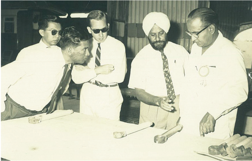
Showing UN Economic Commission for Asia and the Far East (ECAFE) members the new methods of metal spraying in Sentul Railway Workshops to build up worn out piston rods
