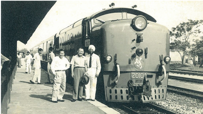
Showing UN Economic Commission for Asia and the Far East (ECAFE) members Malayan Railway Locomotives 20 watt Diesel Electrics that gave balancing problems earlier on
